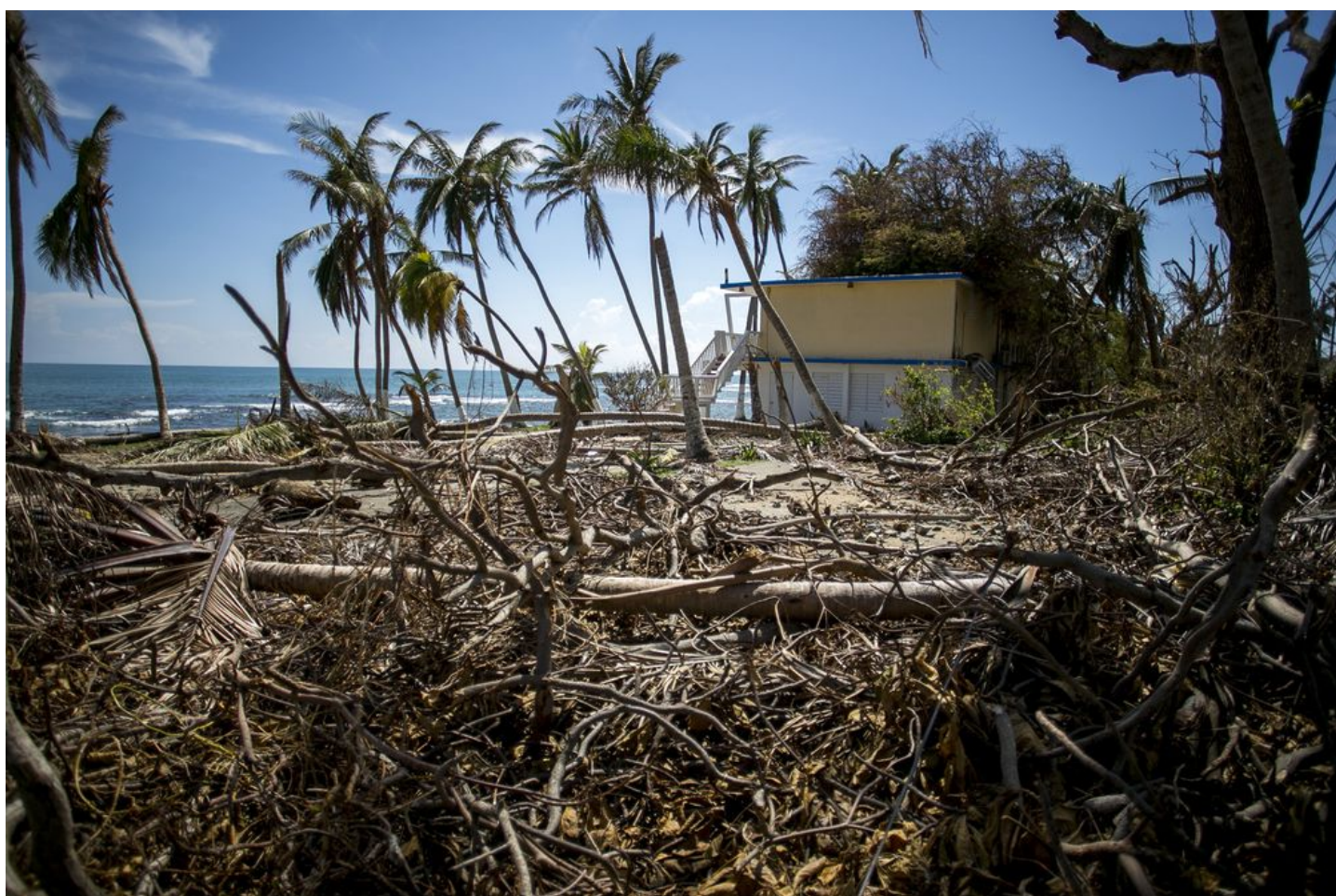
Plant debris sits outside of the damaged Caribe Playa Beach Resort after Hurricane Maria in Patillas, Puerto Rico, on Oct. 6. Photographer: Xavier Garcia/Bloomberg
